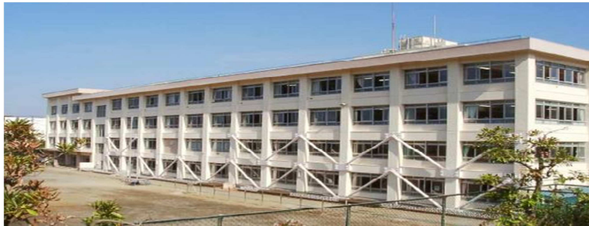
Fig. 1. Application of friction devices [15]
